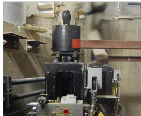
Theater stage lift
